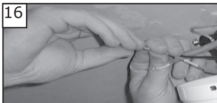
16 Make wire connections to power source using wire nuts provided. Make sure that no filaments are outside of the wirenut. After making the wire connections, the wires should be spread apart with the grounded conductor and the equipment-grounding conductor on one side of the outlet box and ungrounded conductor on the other side of the outlet box. The splices after being made should be turned upward and pushed carefully up into the outlet box.
